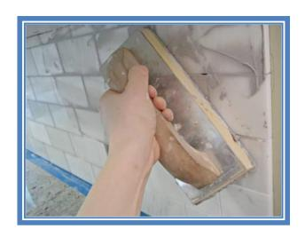
Sanded grout is used where grout lines are 1/8" or wider. Sanded grout has fine sand added to it which keeps it from shrinking too much, unlike the non-sanded variety.
